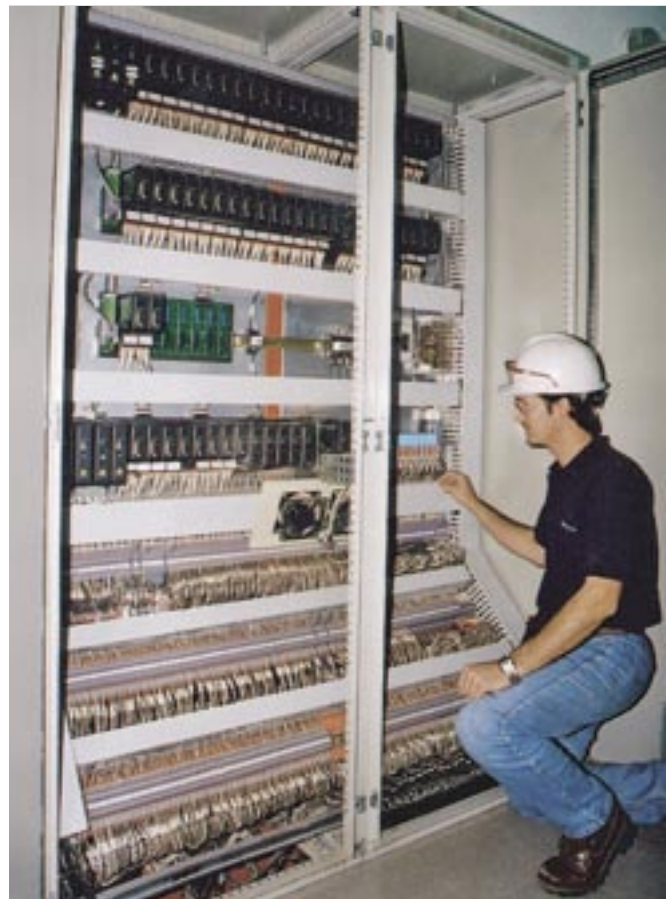
FIG. 6 Field instruments communicate with the digital automation system through modular controllers that can be mounted in field enclosures.
